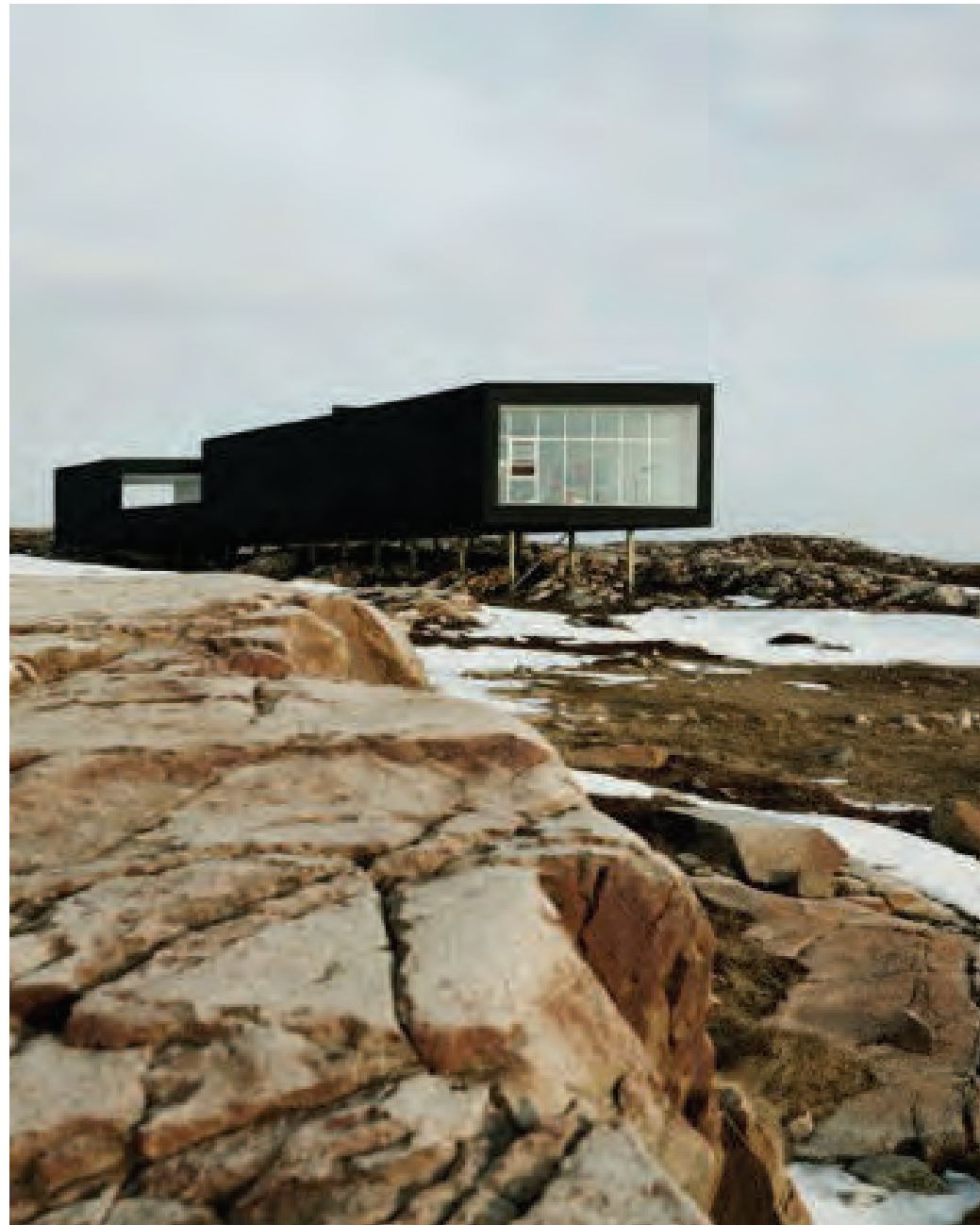
Long Studio / Fogo Island, Newfoundland, Canada / Saunders Architecture
