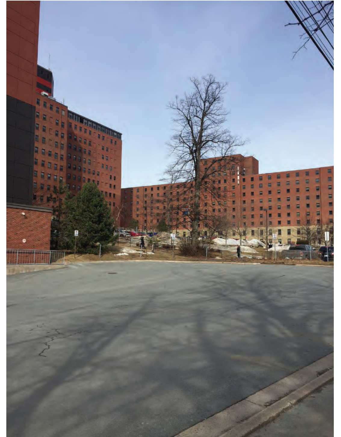
Looking north at Bethune Building
