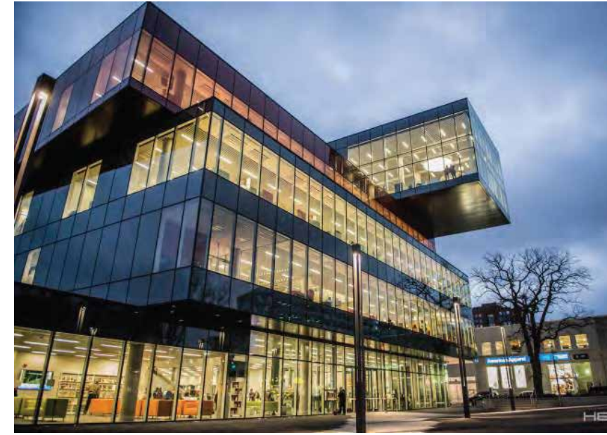
Halifax Central Library/ Halifax, Nova Scotia/ Fowler, Bauld & Mitchell in collaboration with Schmidt Hammer Lassen Architects
