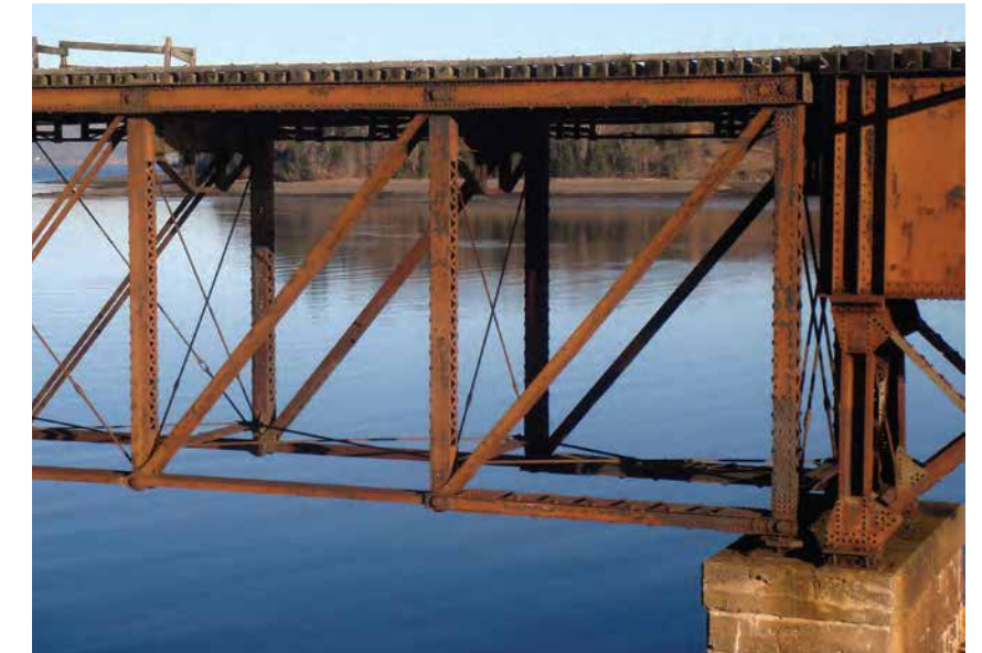
Bear River Bridge / Digby County, Nova Scotia
