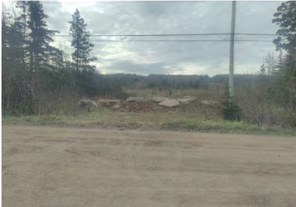
Photo 6. Berm reinstated after drilling completed (May 11, 2022).
