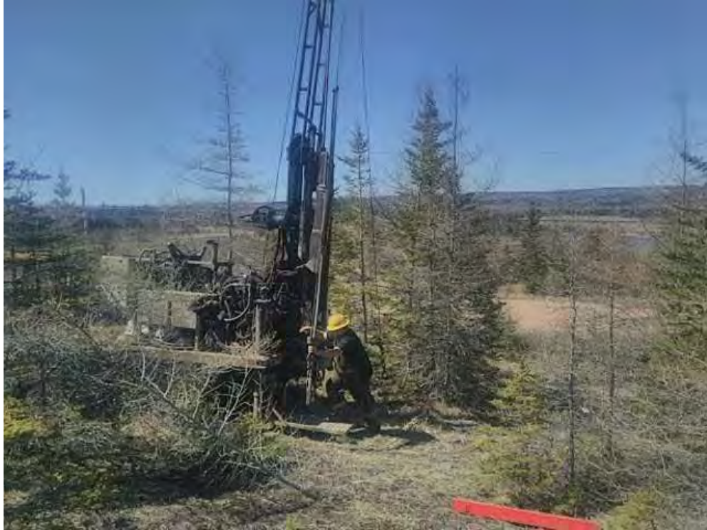
Photo 3. Drilling of MW2, facing west towards Loch Lomond Road (May 10, 2022).
