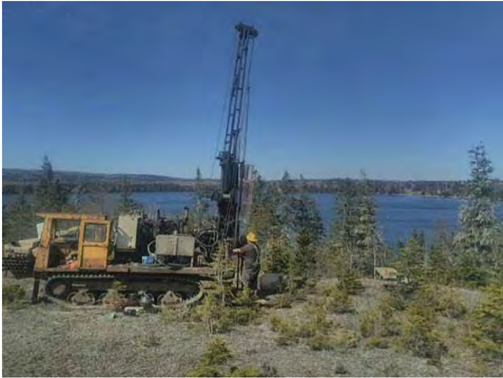
Photo 1. Drilling of MW5, facing north (May 9, 2022).
