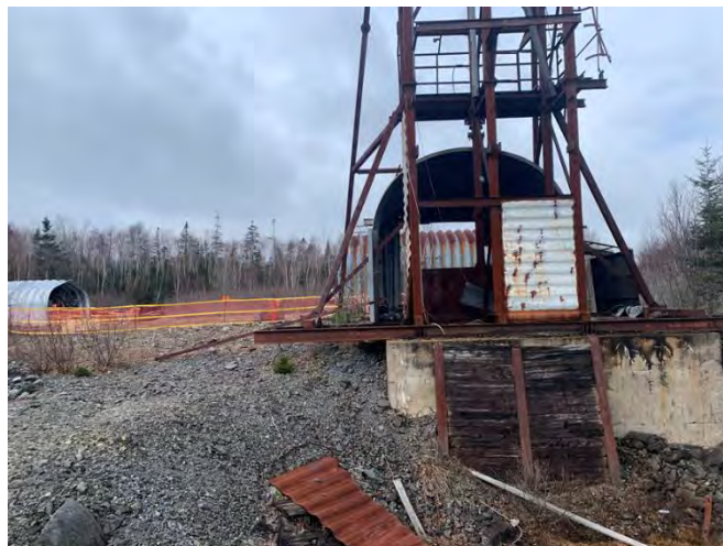
Photograph 8: View of potential headframe over a former mine shaft
