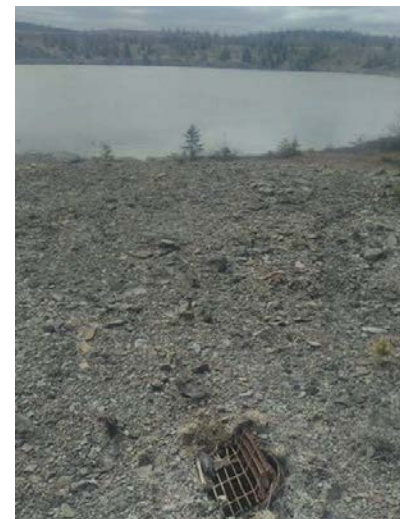
Photo 20. Vertical drain north of APEC 6 (May, 2022).
