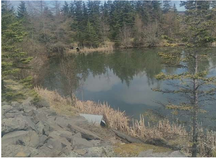
Photo 13. Culverts in APEC 7 (May, 2022).
