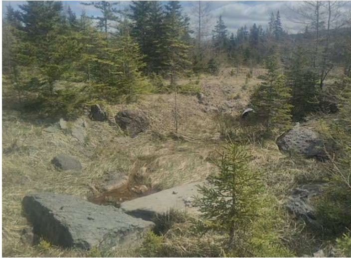
Photo 9. Culvert between APEC 6 and APEC 7 (May, 2022).
