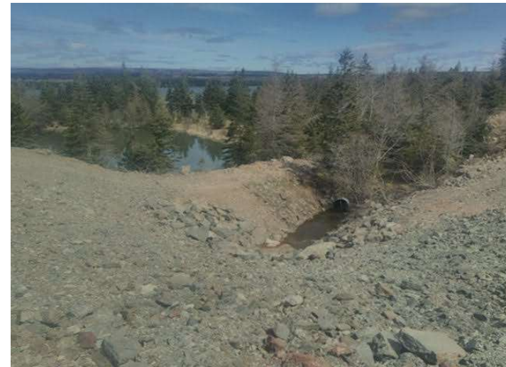
Photo 12. Culvert southeast of APEC 7 (May, 2022).
