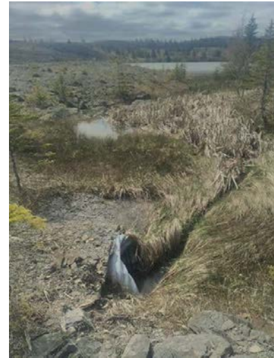
Photo 10. Culvert northwest of APEC 6, running east to west (May, 2022).
