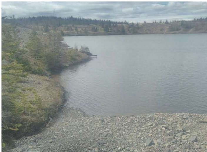
Photo 11. Culvert on east side of APEC 6 (May, 2022).
