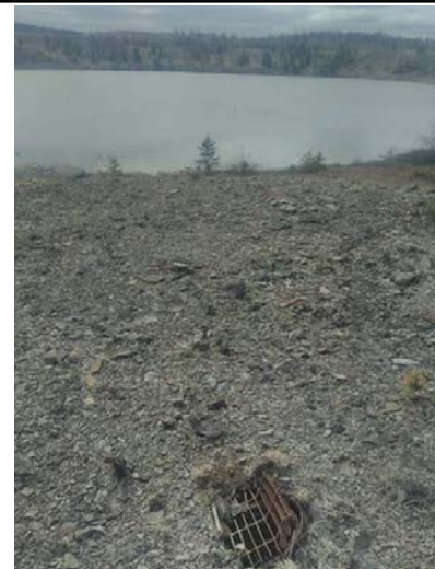
Photo 20. Vertical drain north of APEC 6 (May, 2022).
