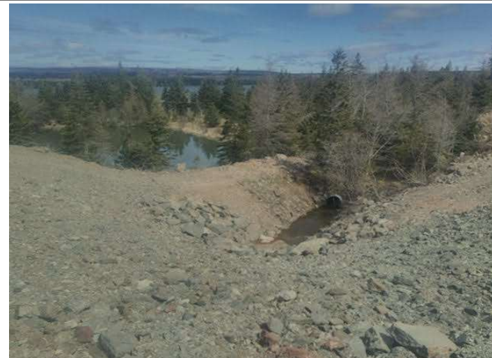
Photo 12. Culvert southeast of APEC 7 (May, 2022).
