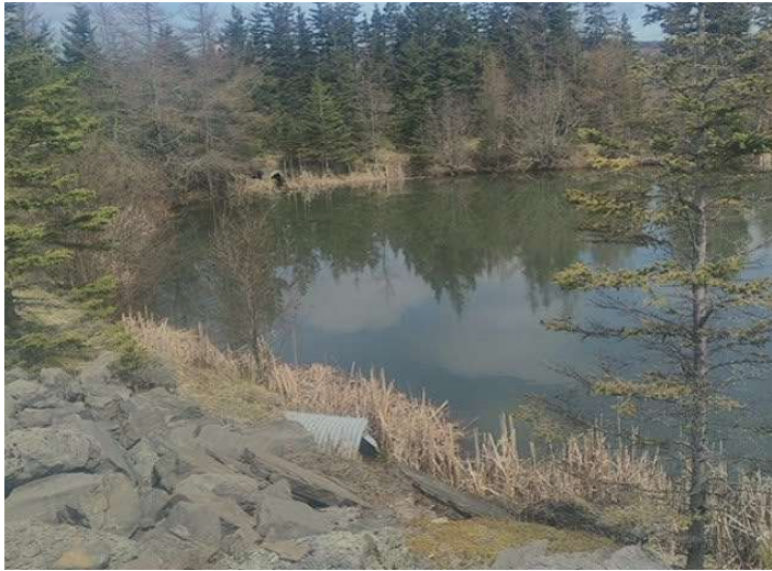
Photo 13. Culverts in APEC 7 (May, 2022).
