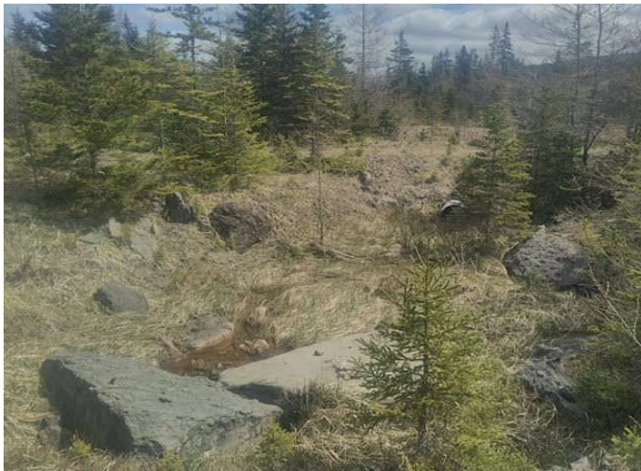
Photo 9. Culvert between APEC 6 and APEC 7 (May, 2022).
