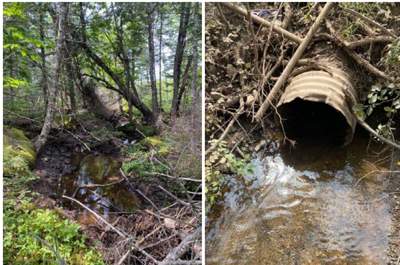
Photos: Photos of WC4 showing upstream (left) and downstream (right), July 26, 2023.
