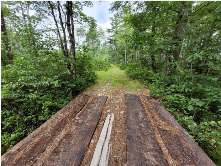
20230720_113100_access road_watercourse crossing_1 km east
