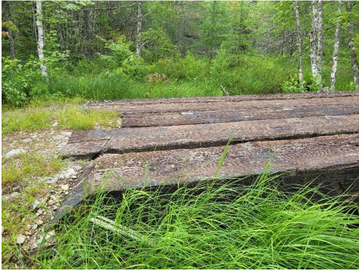
20230720_112443_access road_watercourse crossing_1 km east
