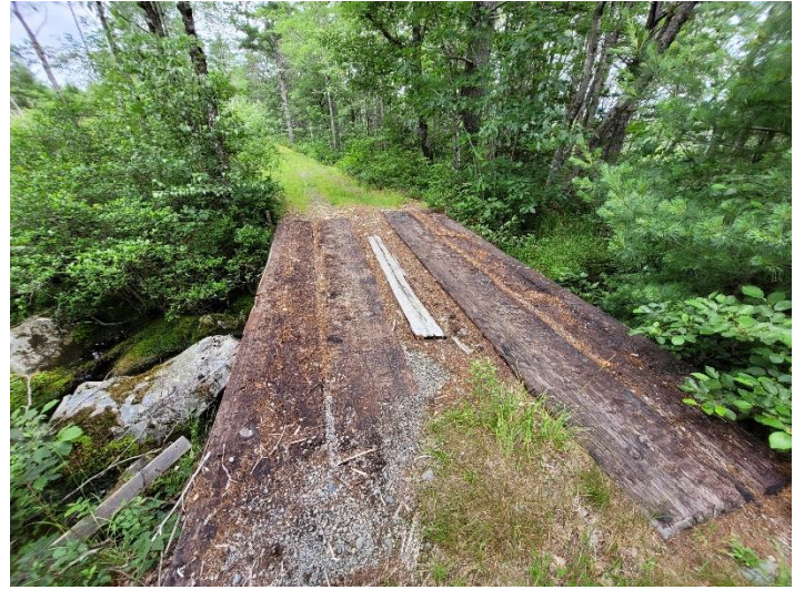
20230720_113048_access road_watercourse crossing_1 km east
